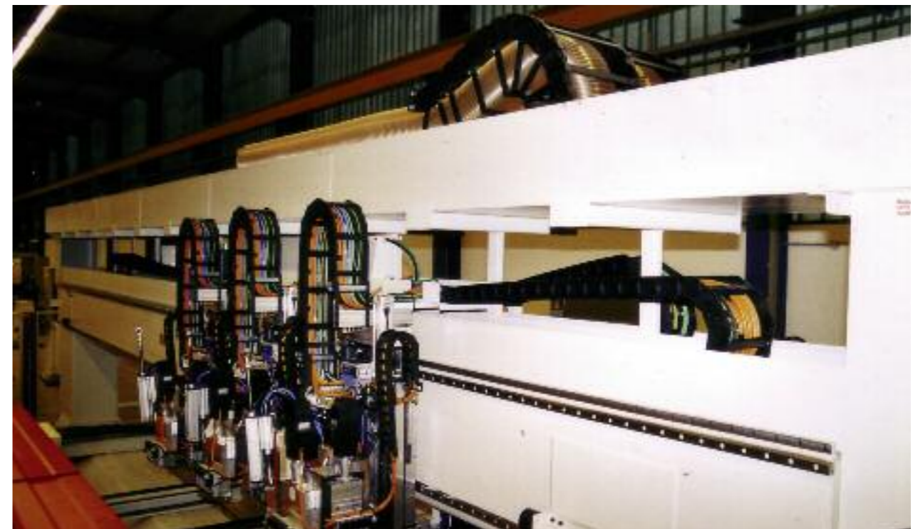
Woodworking machines with e-chains® and chainflex® cables
