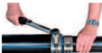
Tighten the locking bolts alternately with a torque wrench to the final torque rate indicated on the label of the connector.
