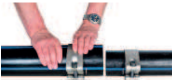
Slide the connectors over both pipes.
